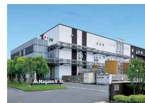
Okayama Plant I
